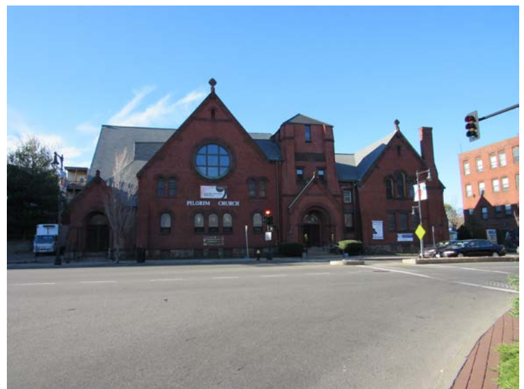
Pilgrim Congregational Church, 544 Columbia Road (1888-1892), view west.
