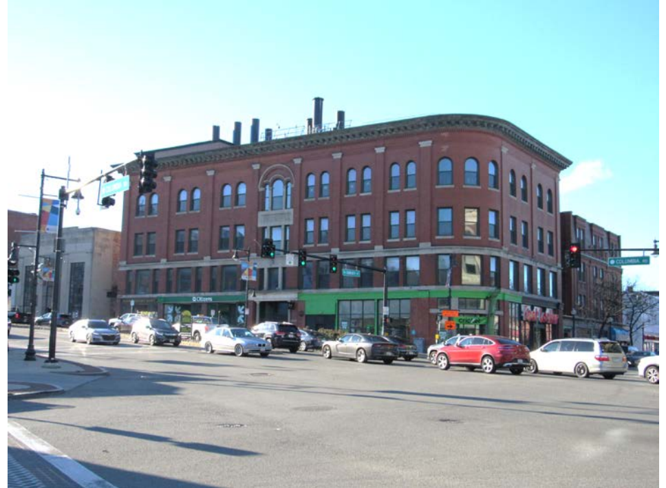
Columbia Square Building, 779-781 Dudley Street / 578-588 Columbia Road (1901-1902), view west.
