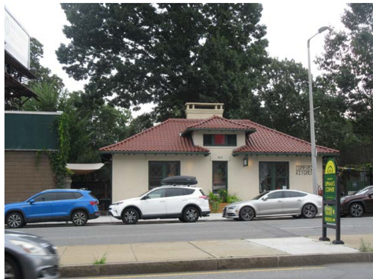
Comfort Station, 611 Columbia Road (1912), view east.
