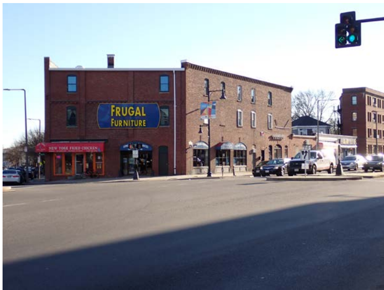
Columbia Road Stables, 523–531 Columbia Road (1880 / 1897 / ca. 1905), view southeast.
