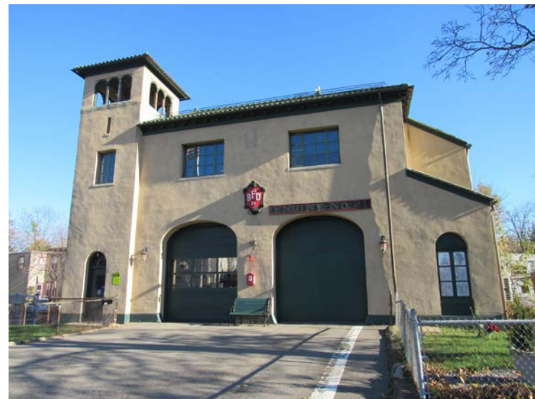
Boston Engine House #21, 643 Columbia Road (1925), view east.
