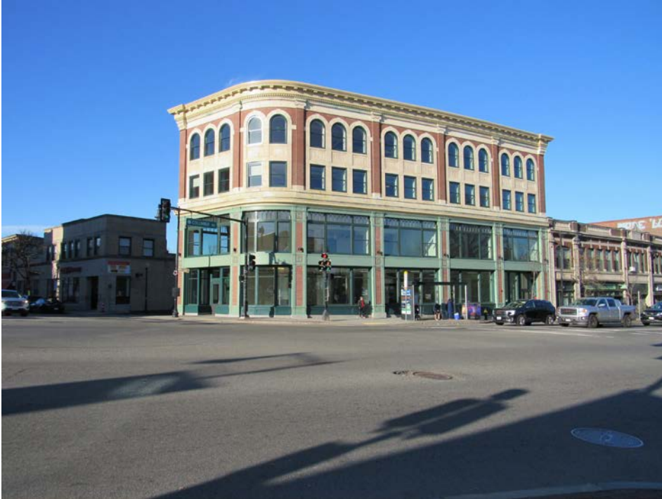
S. B. Pierce Building, 592-598 Columbia Road (1901), view northwest.
